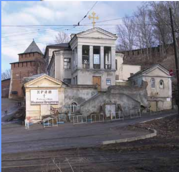
The square of National Unity before and after reconstruction
